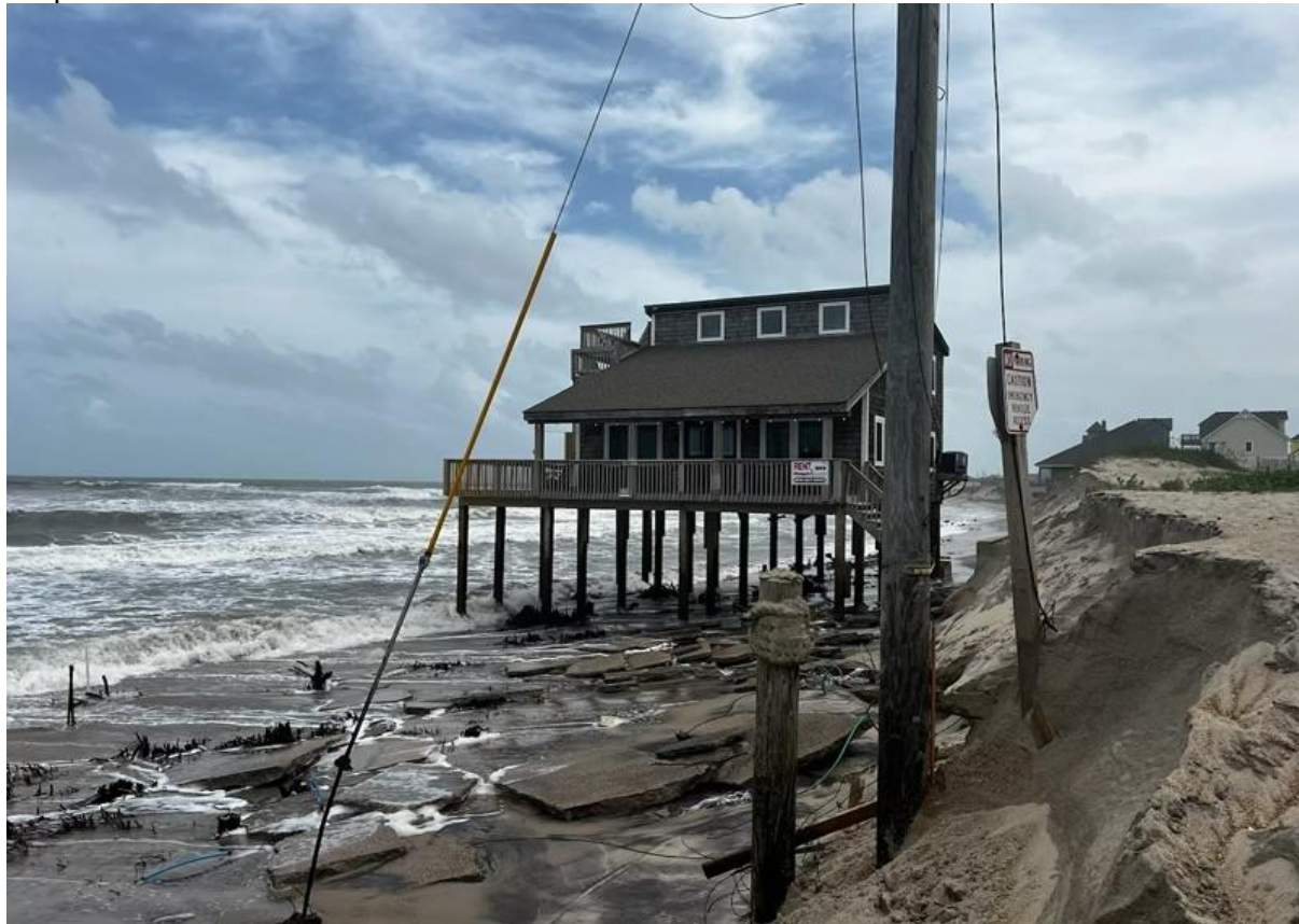
Damaged piling and debris
