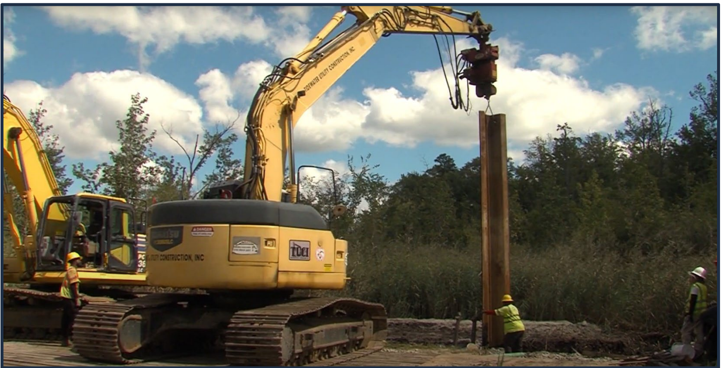
Utility Installation along Centerville Turnpike
